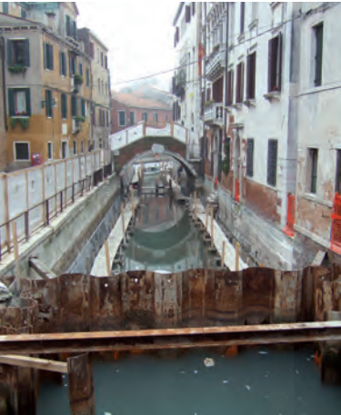
© Unofeld781 / Dredging of a canal with repair of the embankment walls
