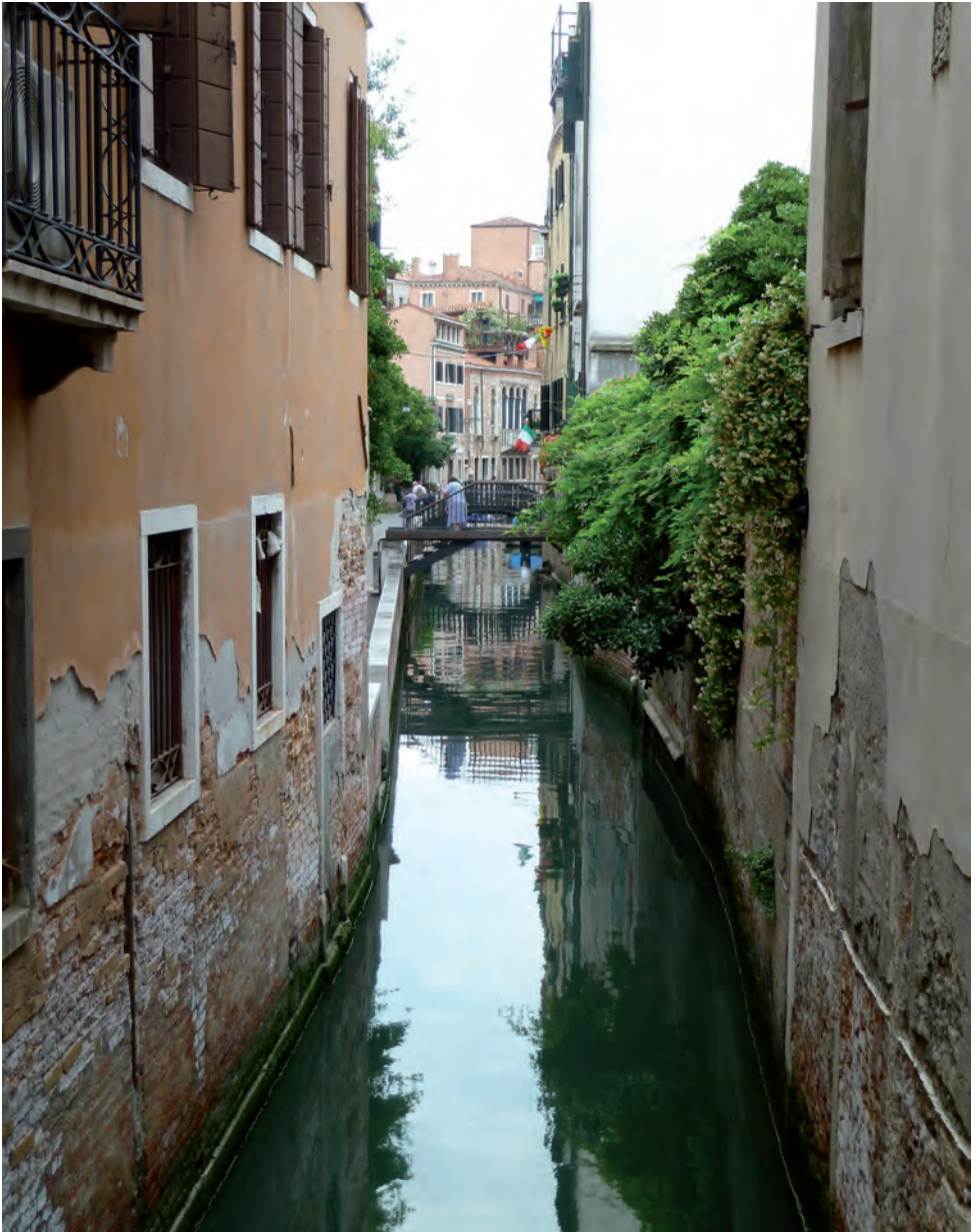
© Abxbay - Rising damp damage to brickwork and masonry. Rio de la Frescada
